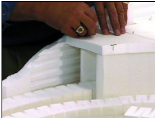
Foam Sheets may be used to form tunnel walls and ceilings.
