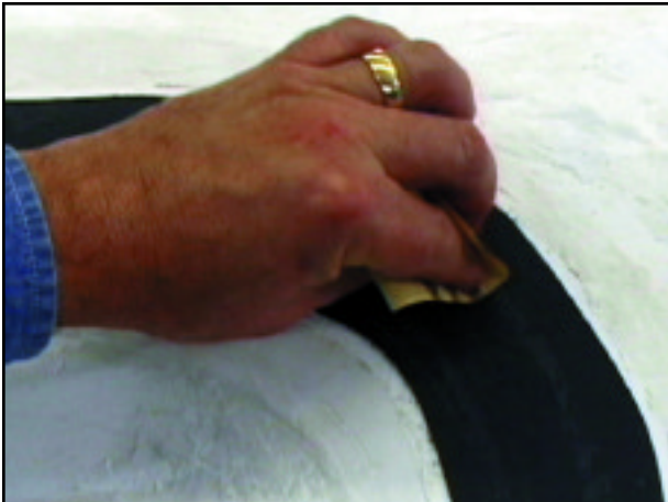
For streaks and scratches, use 220 grit sandpaper.
