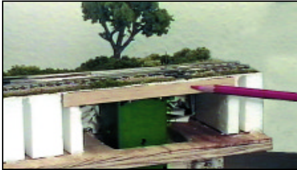
Use a piece of hardboard to support your switch machine as shown in module above.
