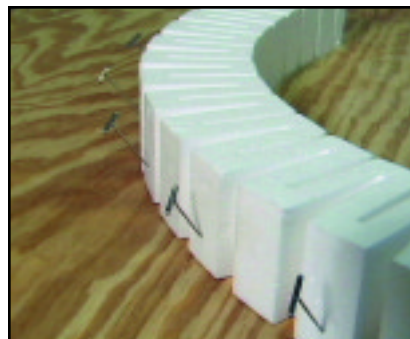
Temporarily pin the Risers to base with Foam Nails.
